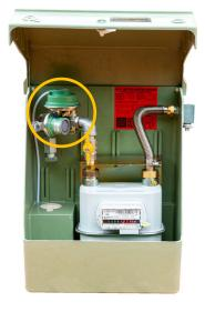
This regulator is used in all medium pressure meter box assemblies supplied by Clesse UK.
